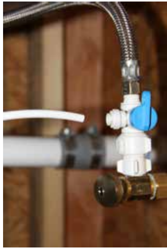
Angle Stop Adapter or T Valve installed at source water.
